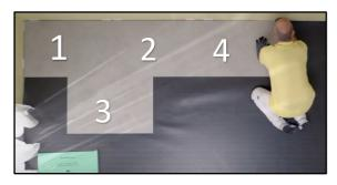
4. Take a third, complete tile (n°4) and click it into the short side of the second tile (n°2). Again make sure the tile is completely in line with the other tiles. Place a placeholder on the long side of the second (n°2) and third (n°4) tile of the first row.
