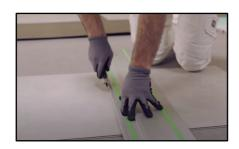
7. Draw the measured distance on a new full tile starting from the top edge (decor) on the short side where the tongue is located. Do not include the tongue. Now cut, with the aid of a ruler and a sharp Stanley knife, two or three times over the piece to be shortened. Then turn the tile with the decor side down and break off easily the cut off piece.
