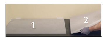
Take a second, full tile (n°2) and click it, at an angle of ±30 degrees, into the short side of the first tile (n°1). Make sure that these are in a straight line with each other. Keep an angle of ±30 degrees when installing all the tiles! This will make the installation a lot easier.
