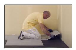
8. Place the piece of tile that is cut in the groove of the last complete tile. The first row of tiles is now complete. Once again, ensure that the tiles remain in a straight line with each other and fix the floor with sufficient spacers.
