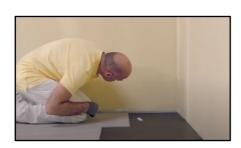
6. The last incomplete tile of the first row should now be fitted. Measure the distance from the top edge (decor) on the short side of the last full tile to a 5 mm distance block, which has been placed against the wall. Caution! Make sure that you do not start measuring from the groove, but from the top edge of the tile!
