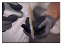
In case of a double pipe, drill a hole with the same diameter as the pipes at all the marked points, adding 15 mm. If the pipes are on the long side of the board, make a 45 degree cut from each hole to the side of the board.
