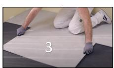
3. Place a tile as a "placeholder" (n°3) on the long side of the first (n°1) and the second tile (n°2). This is not the final position of this tile, but ensures that the first two tiles remain in one straight line. Check that the seams fit tightly.
