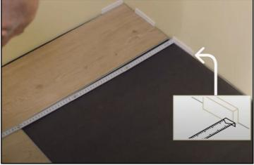
7. From the third row onwards, place the planks row by row. Make sure that you place enough spacers in the expansion joints so that the floor does not shift. Use a varying mix of decors and planks from different packs.
